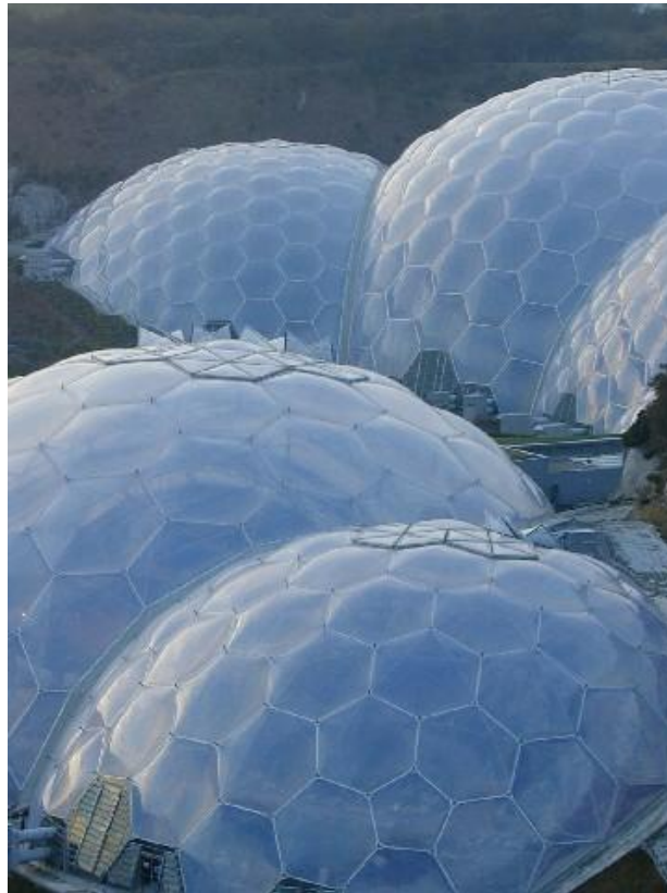
Figure 2. A closer view of the Warm Temperate biome (foreground) and the Humid Tropics biome behind. The inflated pillows with ETFE windows in the curved space frame can be seen with the air input louvres bottom left and some air vents open at the top of the domes.
