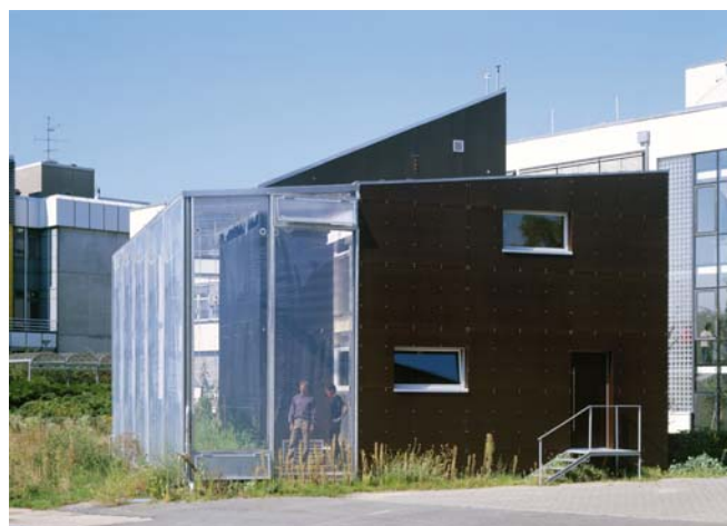
Figure 3. A closed greenhouse attached to a building (Watergy Prototype in Berlin, Germany) which can be used for the direct recycling of grey water and for the concentration of desiccant solutions during summer. The hygroscopic concentrated solution can be stored and be used during winter to absorb water vapour from the greenhouse. The system works as a heat pump, shifting winter greenhouse temperatures to a level, where it can be used for the building's heat supply.
